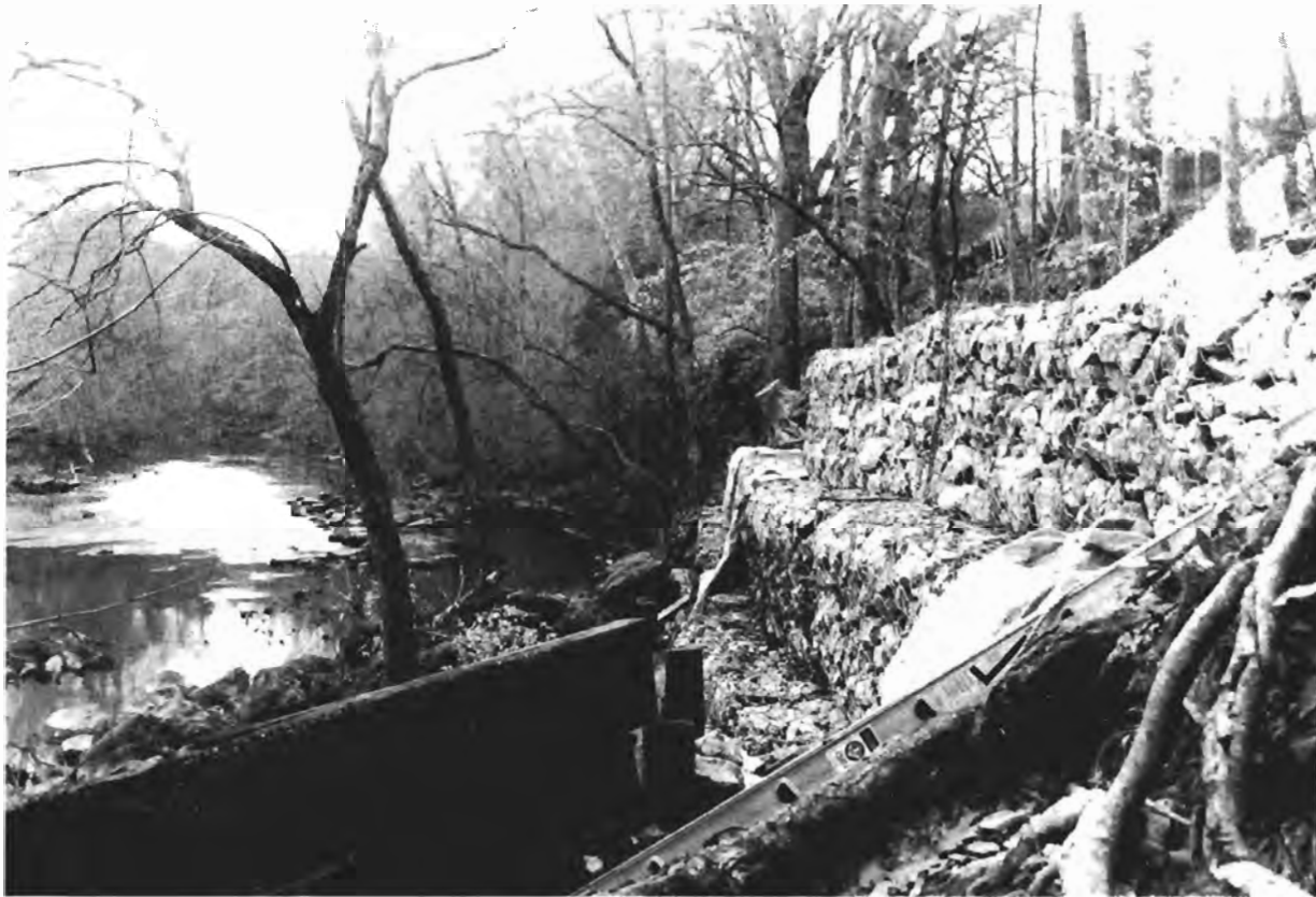
Figure 1. Gabion wall.
