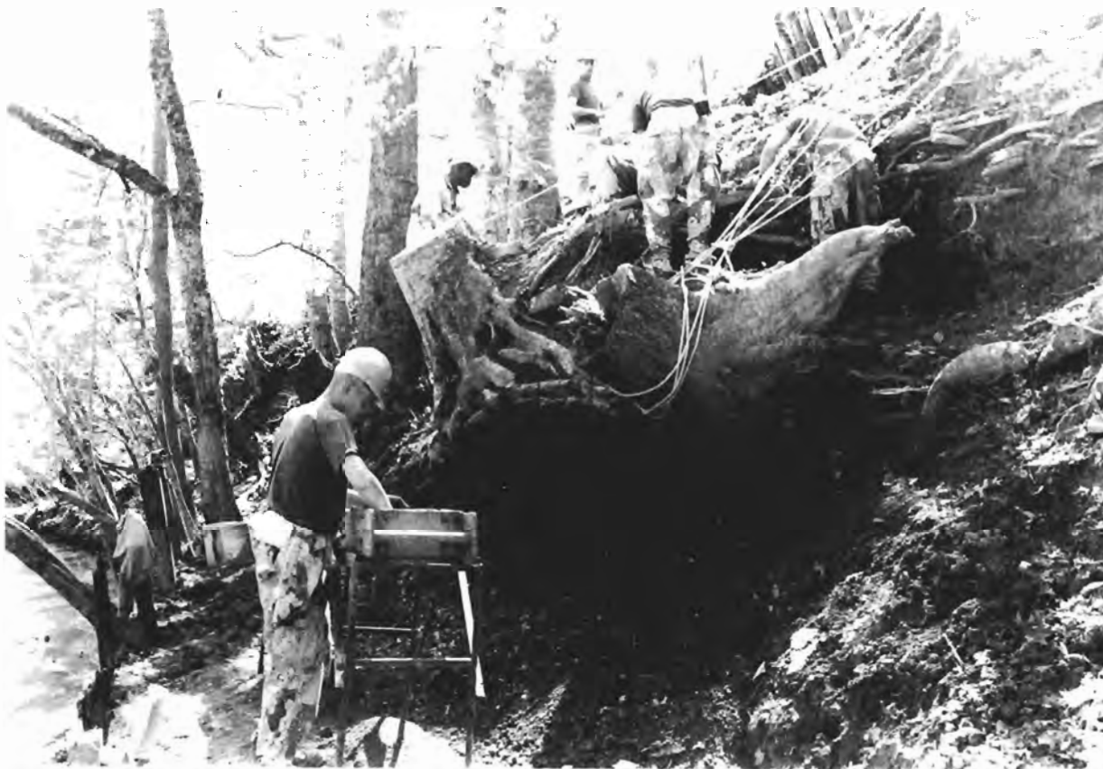
Figure 2. Tree stump removal.
